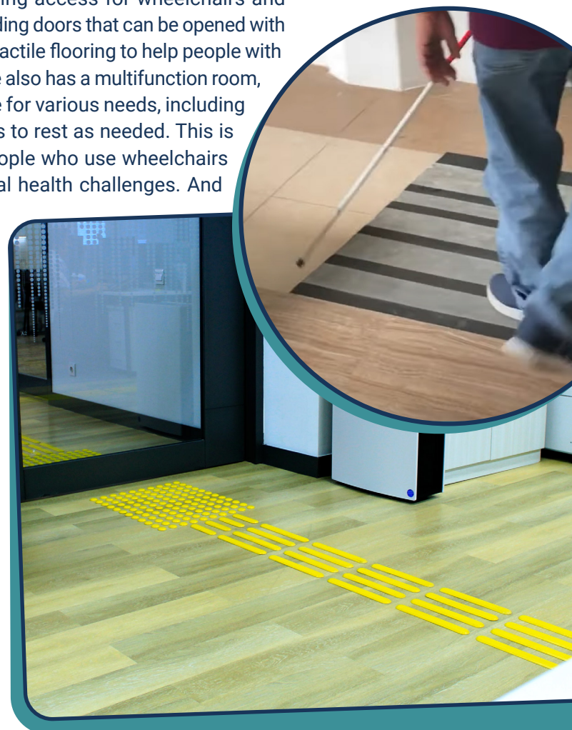
Tactile flooring for people with visual impairments at SKALA's Jakarta office and a ramp for wheelchair users at SKALA's Gorontalo office.
